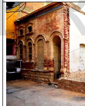
An old stone building demolished by the builders
