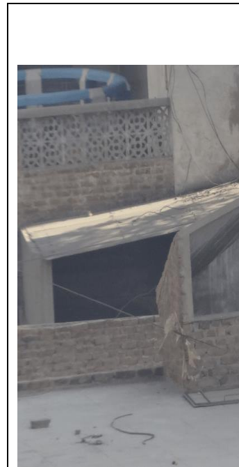
Windcatcher in the house of Hiraabad
